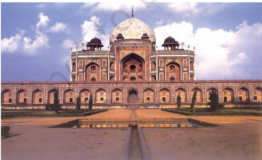
Fig. 11 Tomb of Humayun, constructed between 1562 and 1571. Can you see the water channels?
